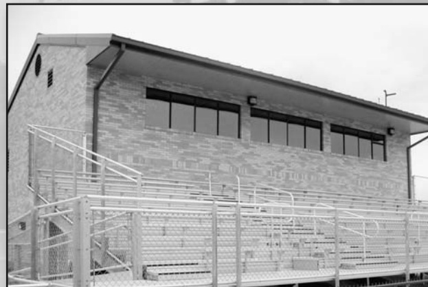
Track & Field moved into a new facility in spring 2004
